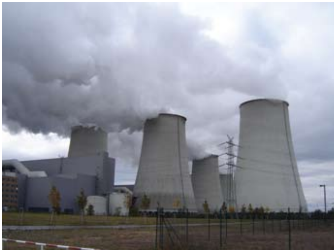
Coal-fired power plant. Photo: Matthias17
